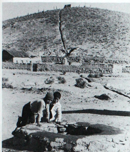
With pipes and a pump from World Vision, water from this well will be transferred to the stone tank atop the distant hill, completing Belén de Andamarca's gravity water system.
